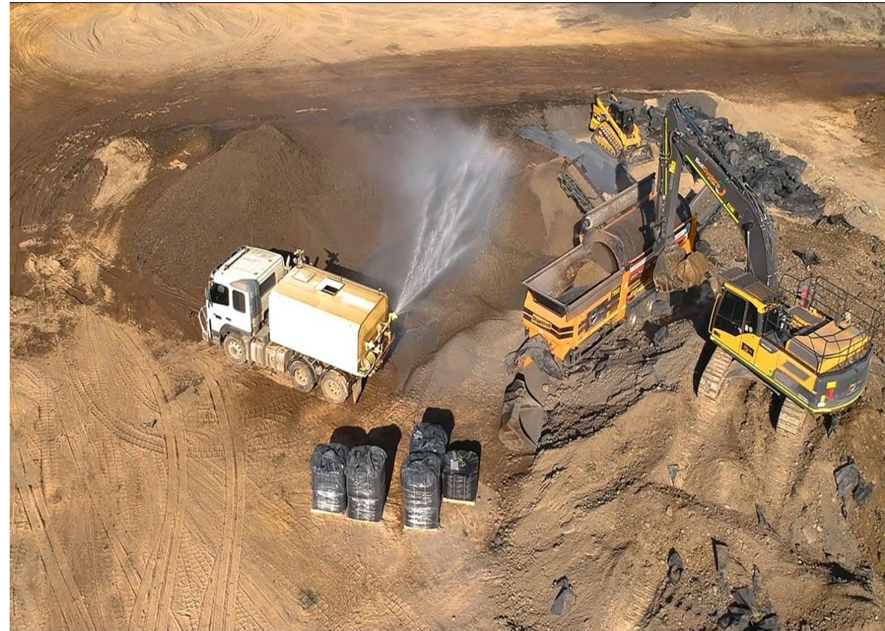
Remediation of AFFF-impacted site (Rembind, 2019)
