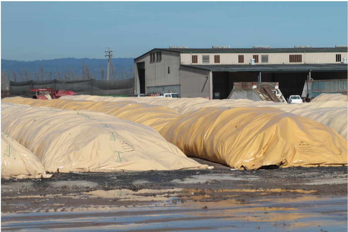
Figure 6. Aerobic Composting for Organics from Mixed Waste System in Gilroy, CA
