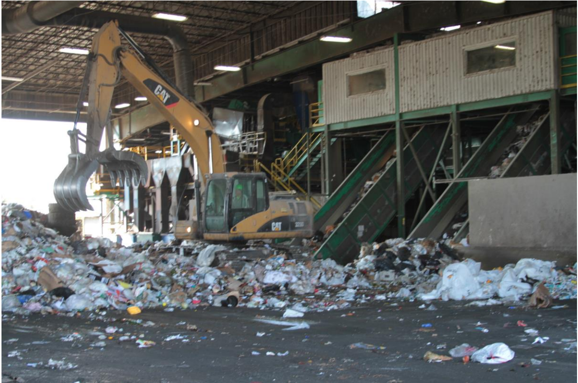
Figure 5. Mixed Waste Processing Facility in Santa Clara, CA
