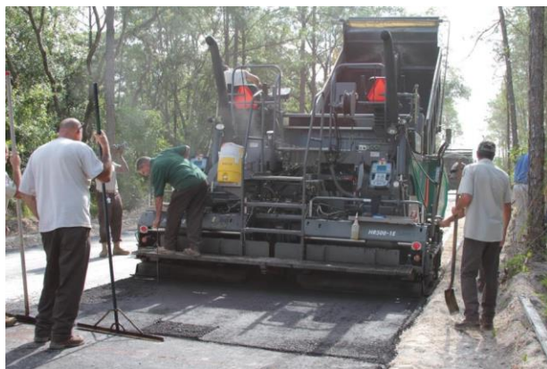
Figure 1: Hot mix asphalt and Portland cement concrete pavements with WTE bottom ash included as a partial aggregate replacement being placed as part of a pilot project at the Pasco County Resource Recovery Facility.
