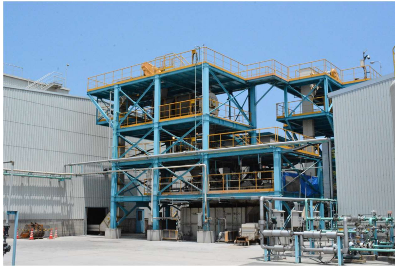
Figure 3. Bottom ash washing system at Mitsubishi Materials Cement Manufacturing Facility Kurosaki Division, Japan.
