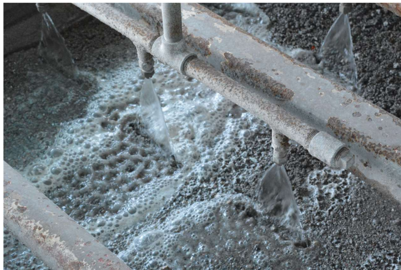
Figure 4. Bottom ash washing system at Mitsubishi Materials Cement Manufacturing Facility Kurosaki Division, Japan.
